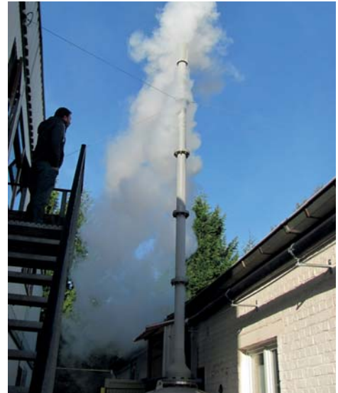
LN2 exhausting line
