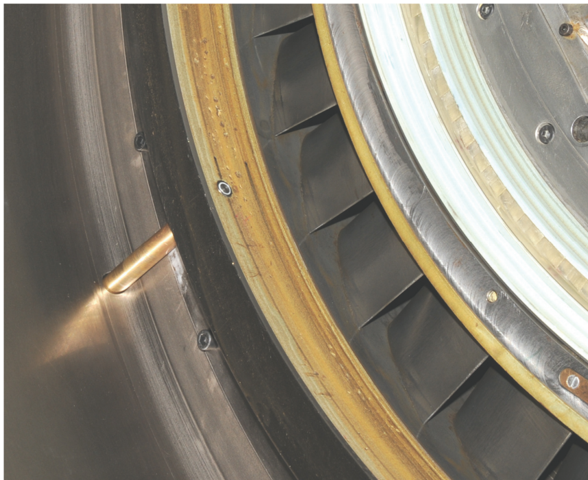
View of the instrumented casing of the high-pressure turbine stage.
